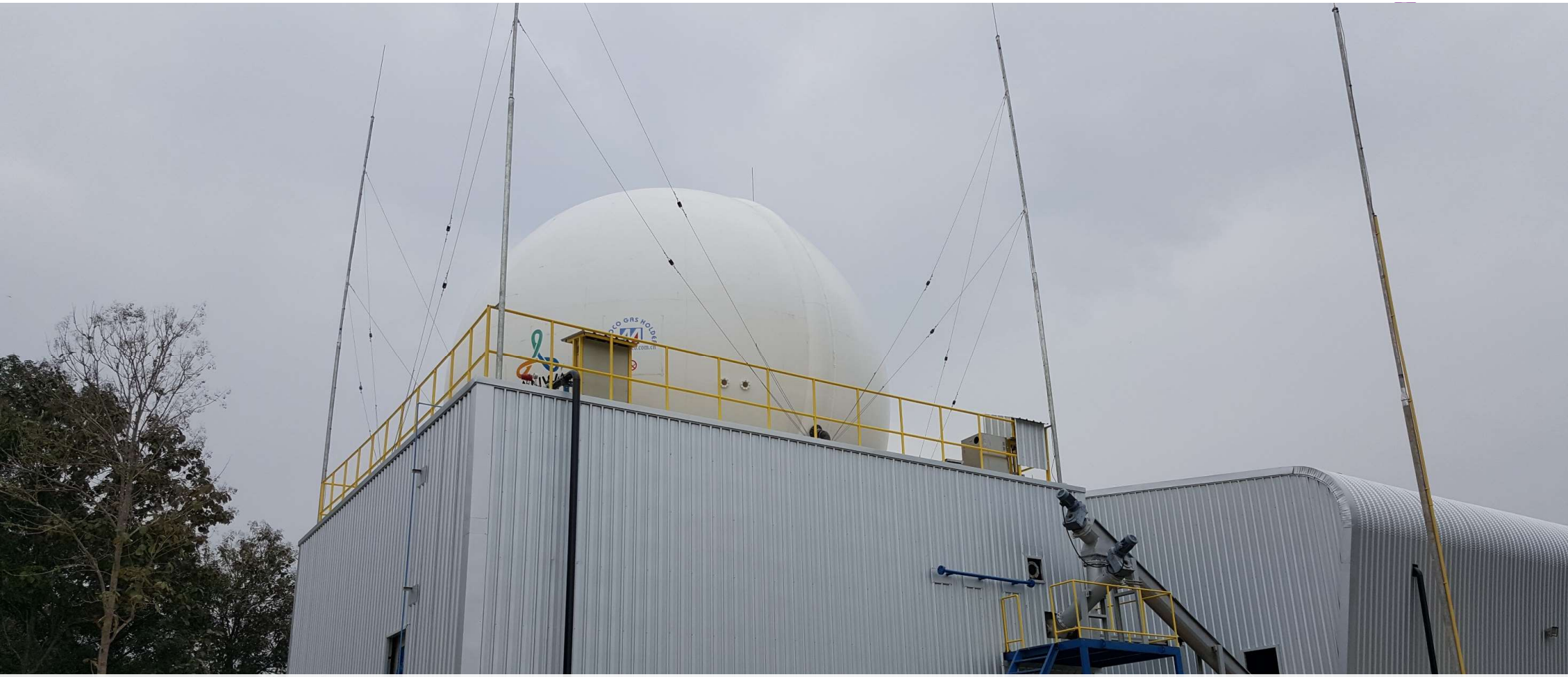
Dry AD Tank
